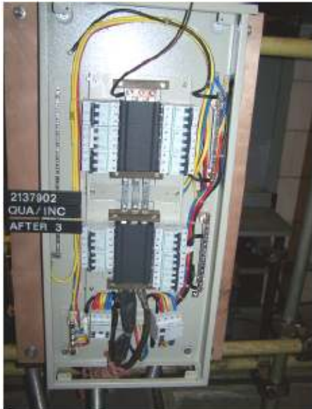
CAMGRO F1 SYSTEM 125A Split type Final Distribution Board Short Circuit Test
