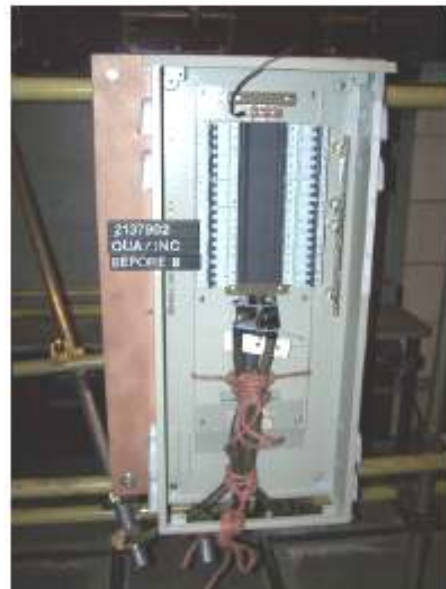
CAMGRO F2 SYSTEM 250A Distribution Board Short Circuit Test
